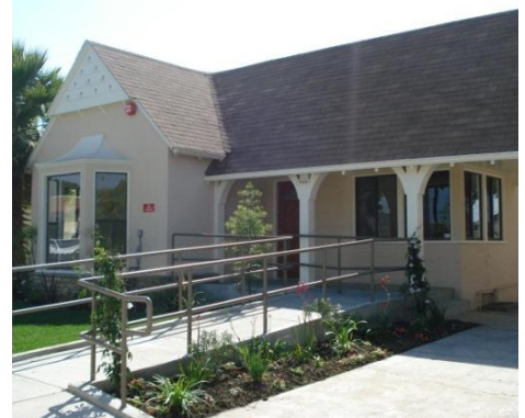
Top: One of the 10 houses renovated for Friend Community Housing
