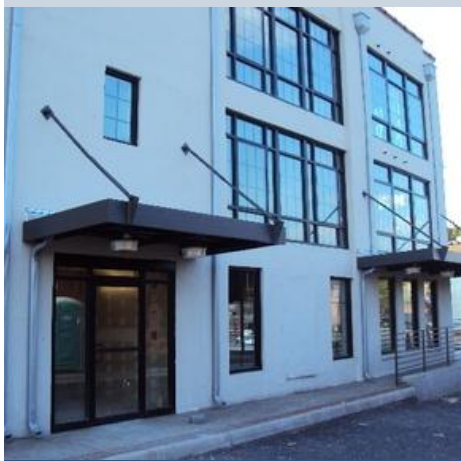
Top: Completed Phase I of Waters Place
